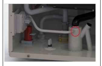
7. Loosen 3 screws on the bottom of the cabinet that holds condensate trap in place.
