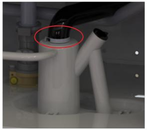
6. Remove hose that connect connected from APS to condensate trap.
