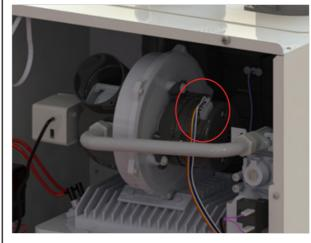
6. Loosen gas pipe nut connected with AGM
