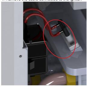
5. Remove two screws to separate ignition transformer from the water heater cabinet.
