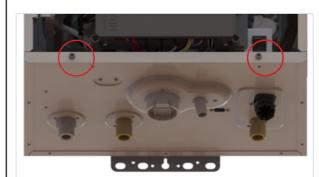
5. Loosen two screws and remove temperature sensor connected with DHW inlet filter.
