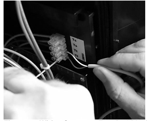
Figure 6 – Wiring Sensor to Terminal Block
