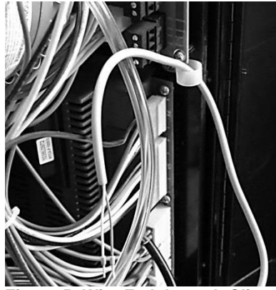
Figure 5- Wire Fed through Clip
