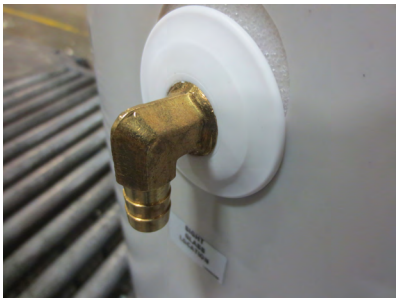
Figure 5 - Brass Drain Back Sight Tube Fitting
