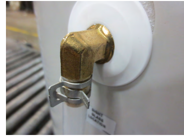
Figure 6 - Sight Tube Secured to Brass Fitting
